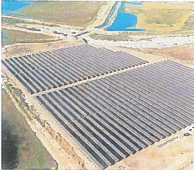
Cawelo Irrigation District (3,500 kWdc)
