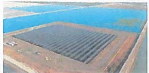
James Irrigation District (1,350 kWdc)
