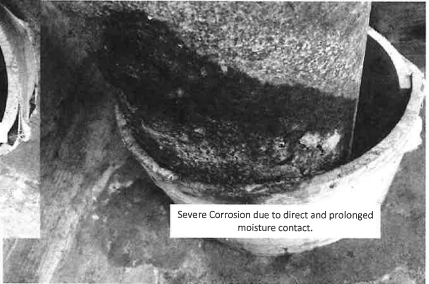
Figure 7 Elkhorn Slough Force Main - Corrosion System-Wide FSP Castroville Community Services District
